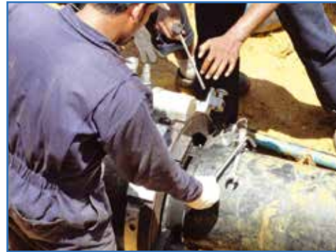
DLW use on-site for gas pipeline contractors
