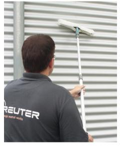
Surface cleaner for cleaning, derusting and passivating large surfaces
