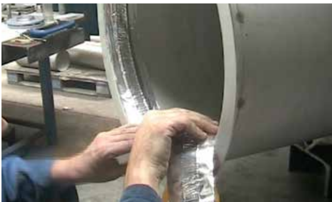
Step 1: Simply stick the tape onto the pre-cleaned weld joint area.
